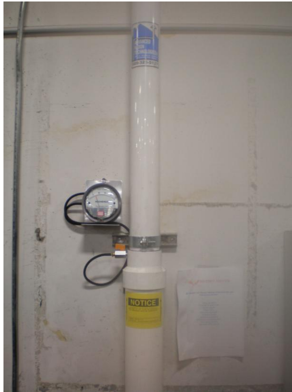
Photograph 1: Riser leading to roof network with gauge.
