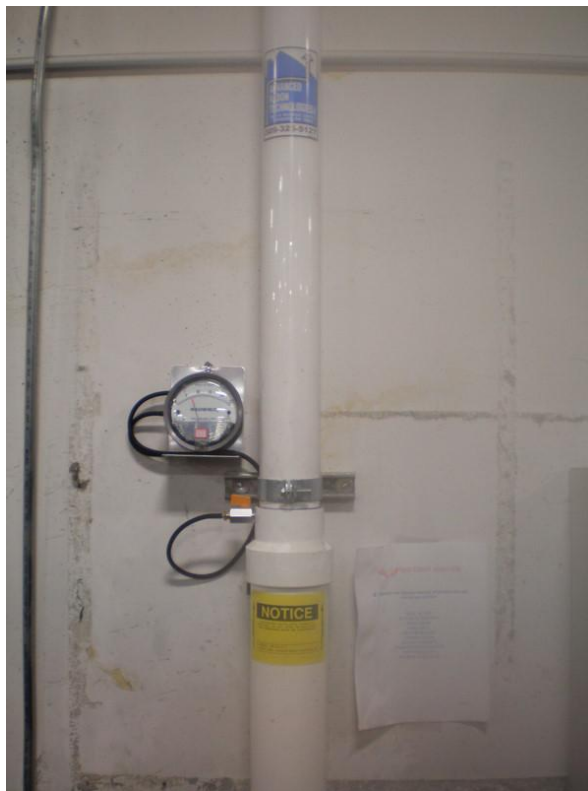
Photograph 3: Depressurization leg and gauge.
