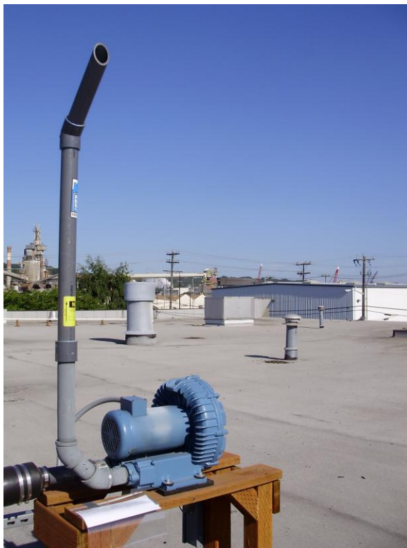
Photograph 15: Blower and stack with nearest air intake in the distance, approximately 36 feet away.
