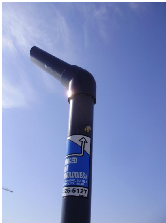
Photograph 16: Stack with air sampling port (plugged).
