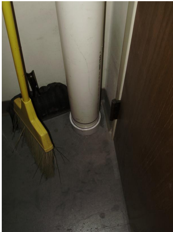
Photograph 2: Visible portion of sump.
