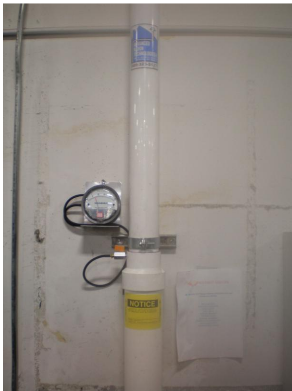
Photograph 4: System gauge and polyvinyl chloride tubing leading to roof network.
