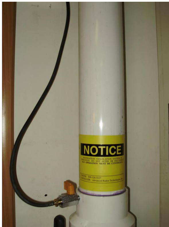
Photograph 5: Pressure hose leading from depressurization leg to gauge.
