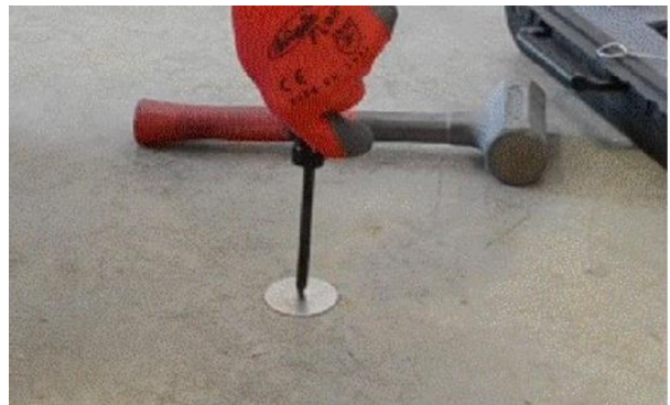
Figure 5. Tightening the Secured Cover
