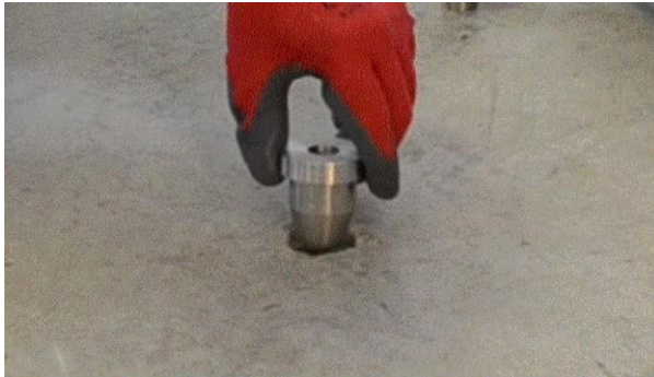
Figure 3. Testing Depth with the Drilling Guide
