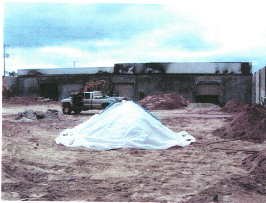
May 21, 2004: Looking W at covered stockpile of suspect soil, N-Stockpile
