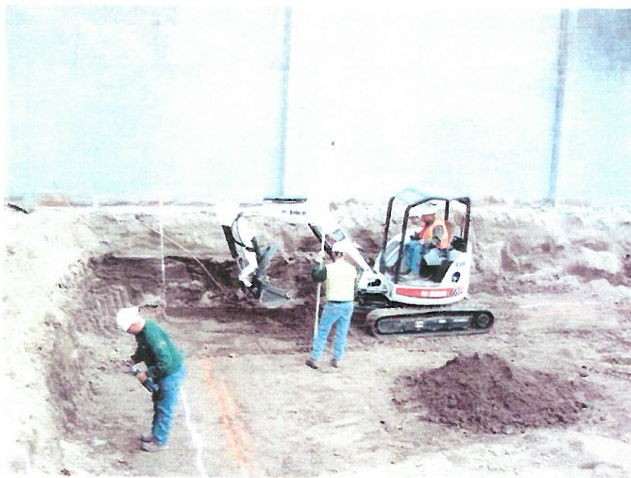
May 20, 2004: Looking N at stormwater vault excavation
