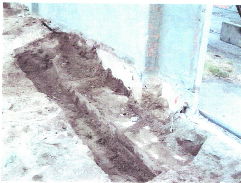
May 21, 2004: Excavated footing along S wall
