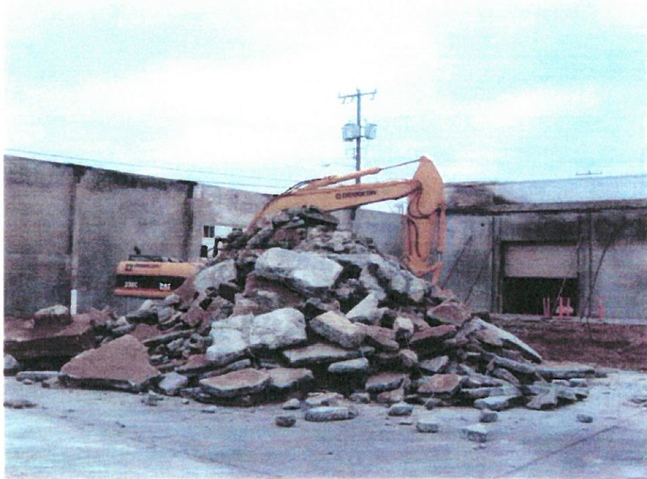
May 11, 2004: Slab removed from the W and SW areas
