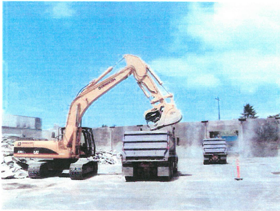
May 12, 2004: Slab removed from W being loaded for off-site disposal
