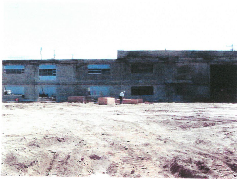
May 24, 2004: Looking E at site with 100 percent of slab removed
