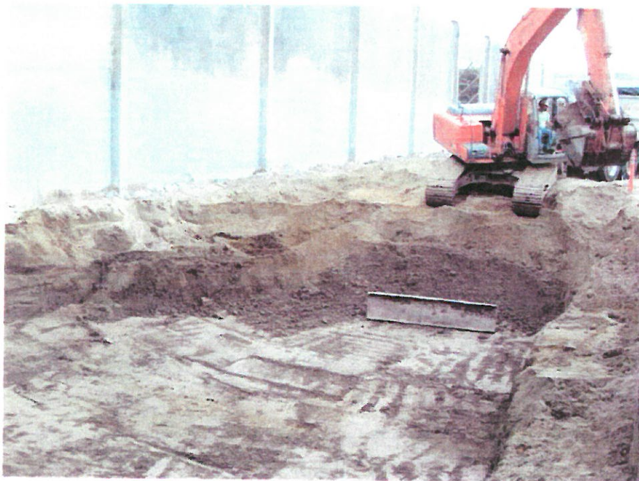
May 19, 2004: Looking E at stormwater vault excavation
