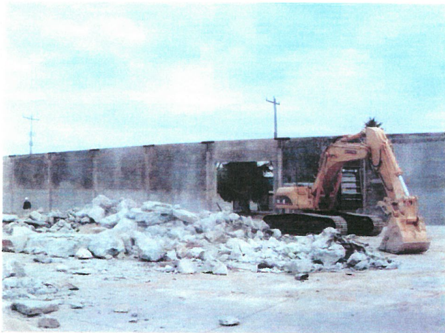
May 17, 2004: Looking N at removed slab and chunks of broken footing
