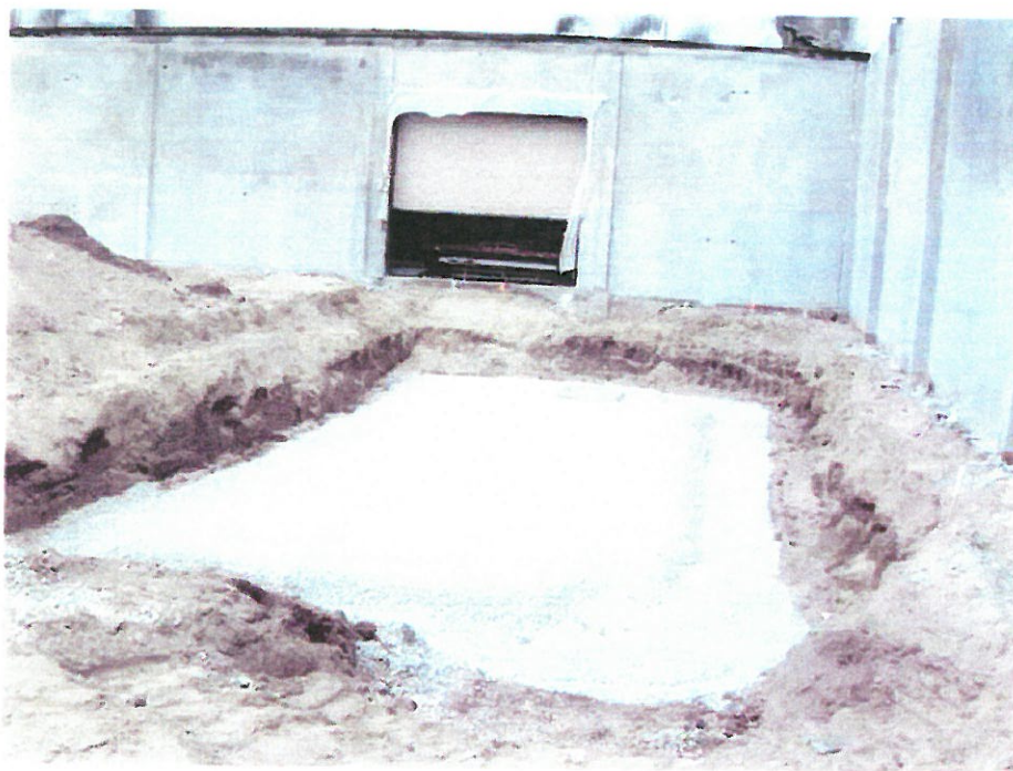
May 21, 2004: Looking W at stormwater vault excavation with bedding material
