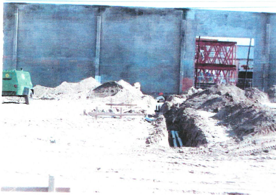
June 9, 2004: Looking S at utility trench in SW area
