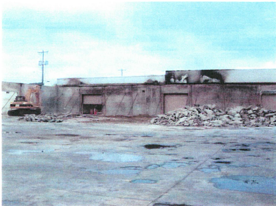
May 11, 2004: Looking W at slab removed from NW and W
