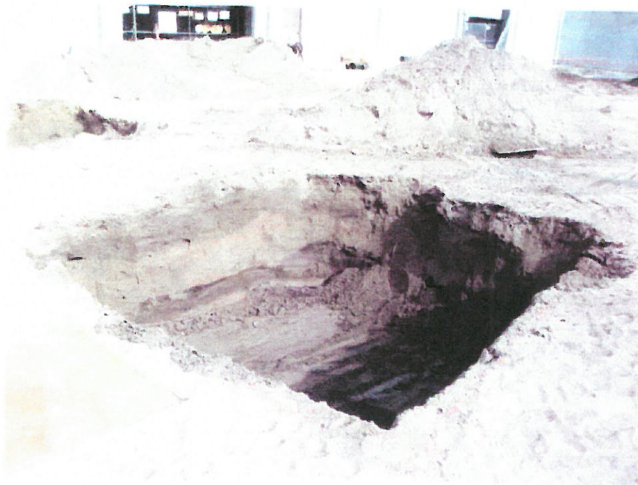
June 8, 2004: Internal footing excavation in SW area
